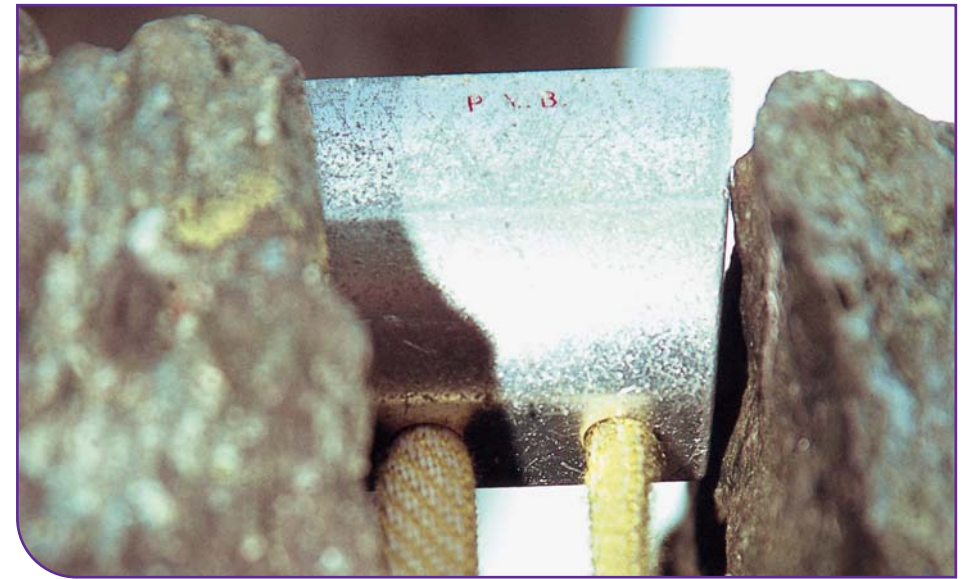
Figure 4.3 An example of poor placement in rock – the nut is not ‘seated’ with all of its edges in contact with the rock
